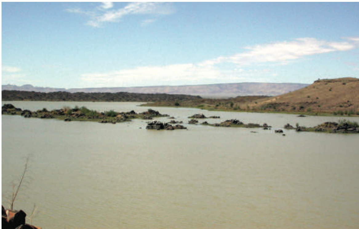
Naute Dam in southern Namibia
